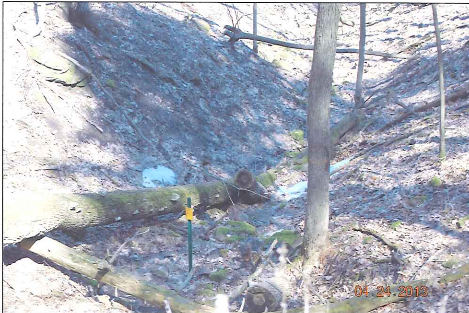
Taken from the Southeast, at fence between Tie #2 & Tie #3
