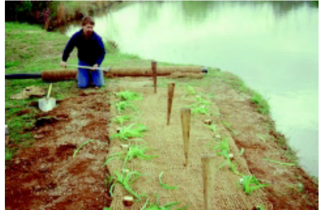
Figure 16-55b Completing installation of reed clump system (Robbin B. Sotir & Associates photo)
