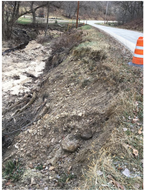
County Highway F, Halls Valley
