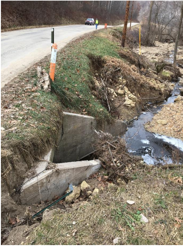
County Highway F, Halls Valley
