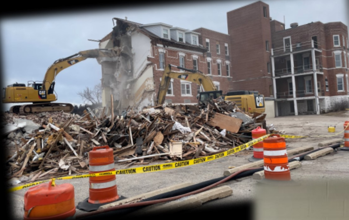
Rolling Hills Building A Demo
