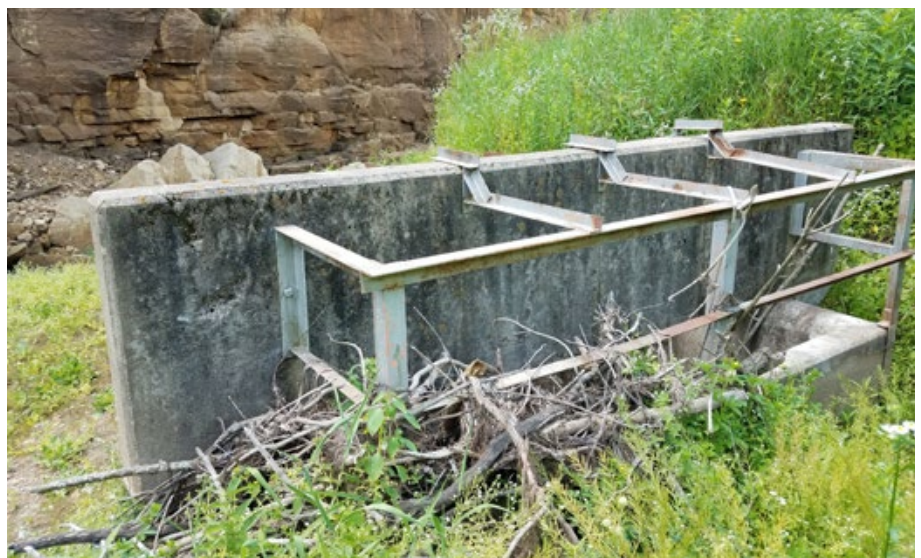
Water inlet at one of the breached dam sites in the Coon Creek Watershed. Photo by Eric Booth
