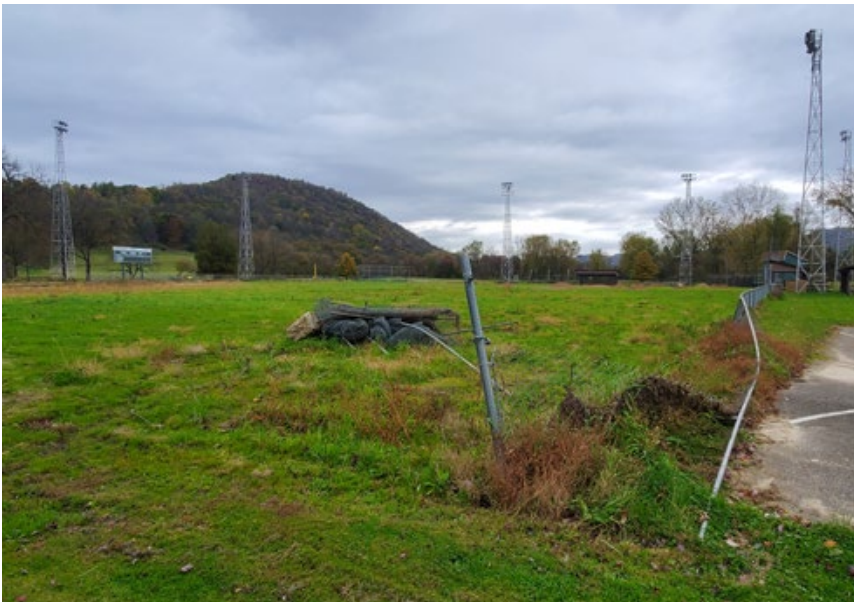
Public park and baseball fields in Coon Valley where repetitive flood damages occur, shown in 2019. Photo by Eric Booth
