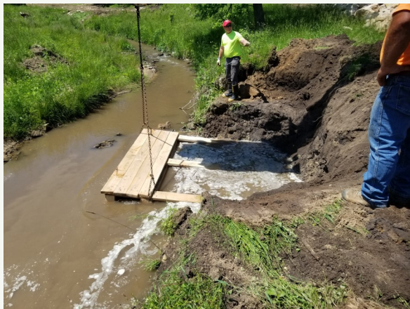
LUNKERS Installation Process
