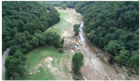
Flood runoff in valley bottoms damages infrastructure and degrades habitat quality for fish and aquatic organisms.
