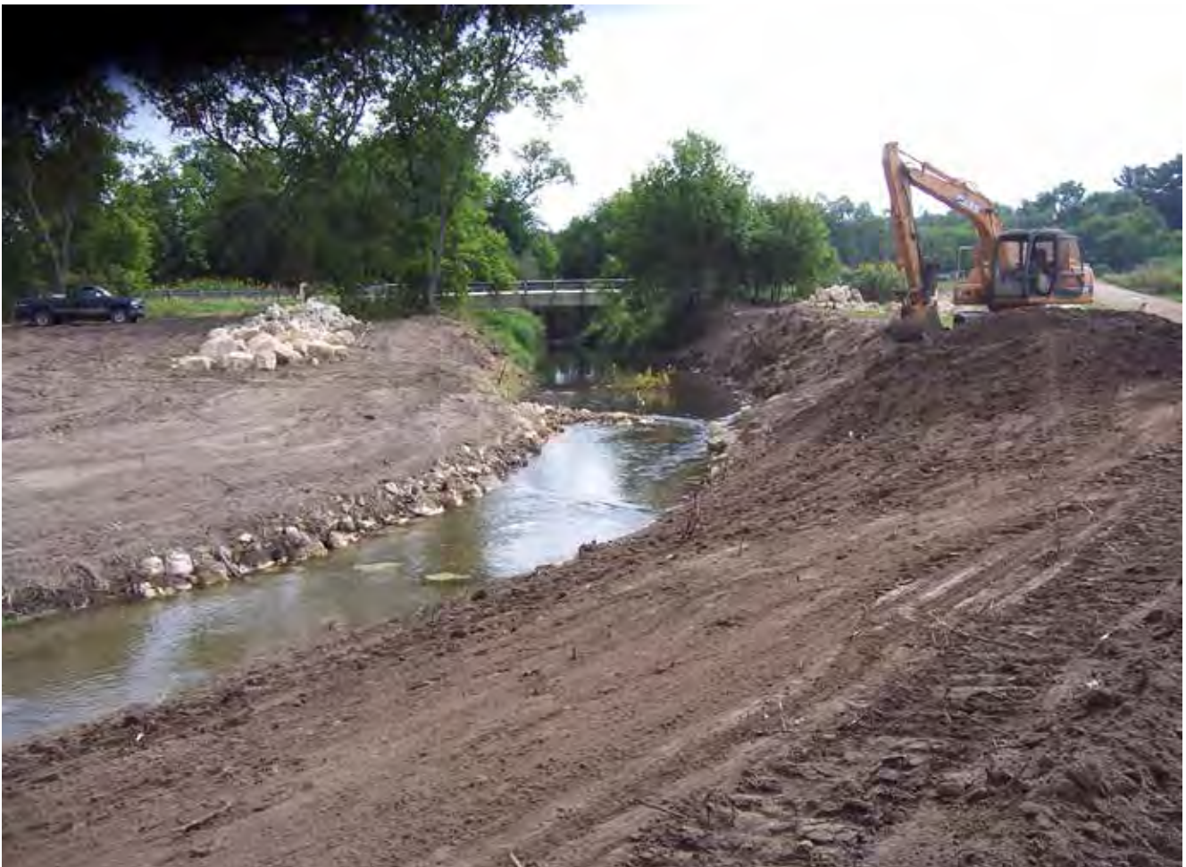
Restoring resilient watersheds can include re-shaping stream banks to accommodate more natural flow patterns.
