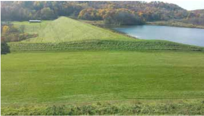
Grass cover can serve multiple purposes - in pastures, with native grasses for wildlife habitat, and as a component of flood control structures.
